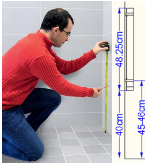
Figure 4.1 Mark the Height of the e Lea™ Activity Sensing Clamps
