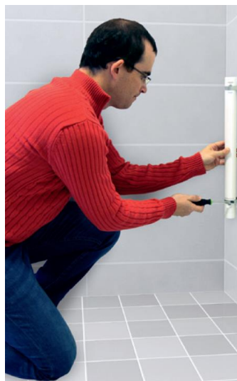
Figure 4.2 Secure the Lower the e Lea™ Activity Sensing Clamp lightly in Place
