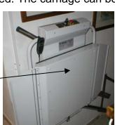
Turn off key switch and lift up the barrier
