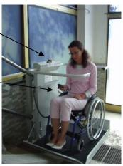
Always watch the stair! If there is danger that the platform drives against an obstacle stop the lift by releasing the directional control button.
